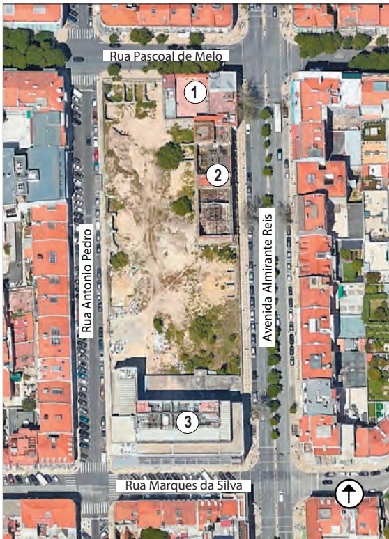
Figure 4: Aerial view of the project site. (source: Google Earth)
