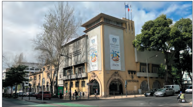
Figure 5: Corner of Avenida Almirante Reis and Rua Pascoal de Melo. The Portugalia restaurant and, on the left, the deteric historic building. (photo: V. del Rio)
